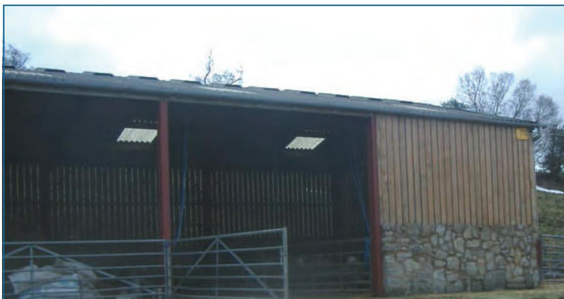
Fig 23: Conspicuous plinth walls should be clad with timber or stone
