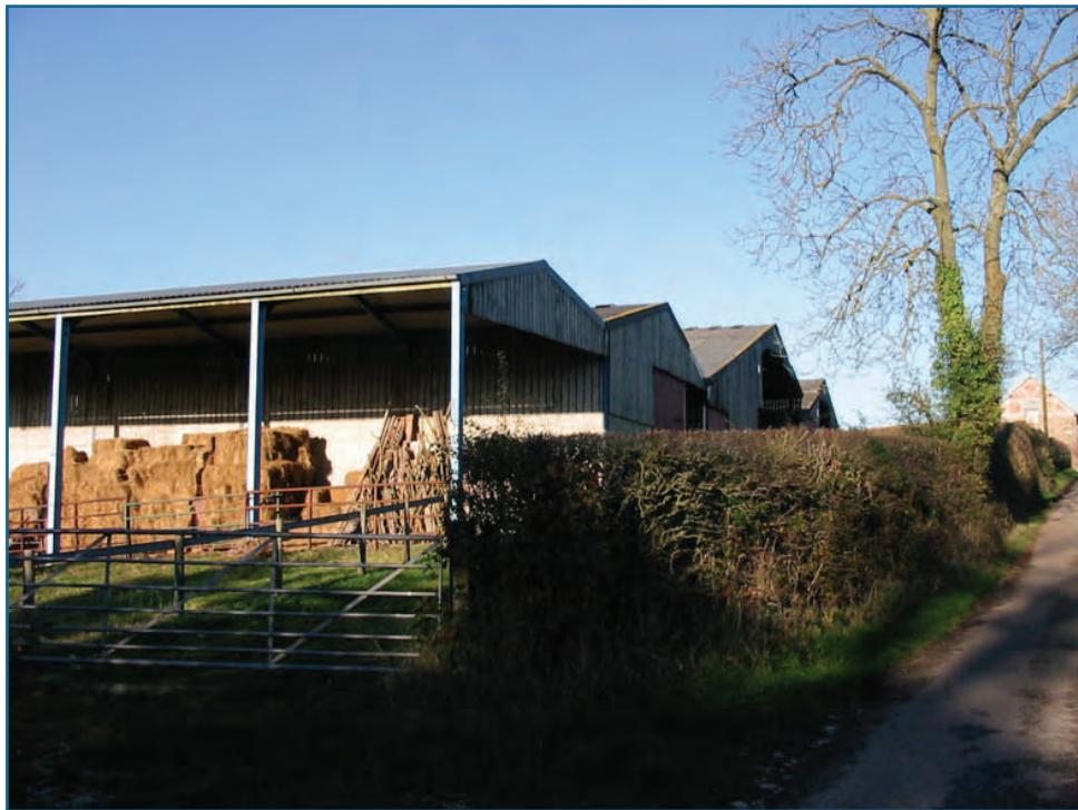
Figure18: Open-sided hay barns positioned next to closed-sided structures to reduce visual impact
