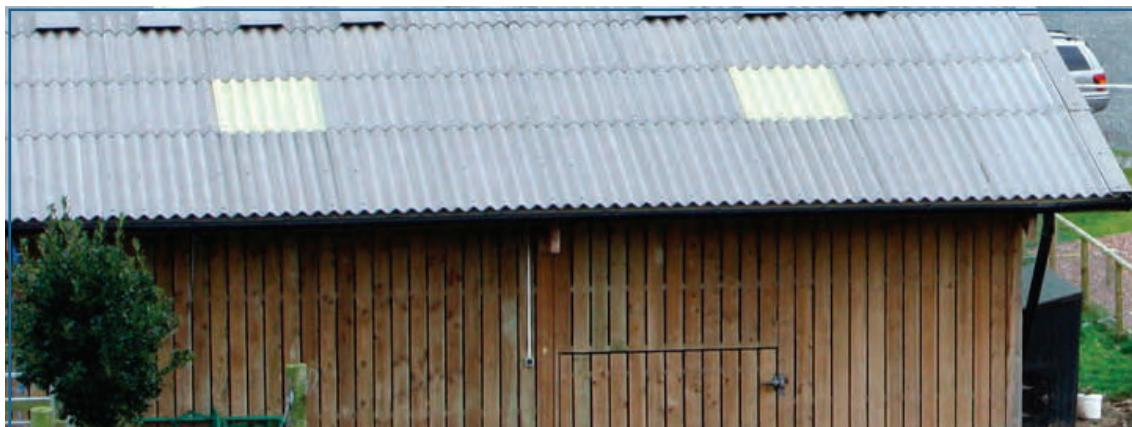
Figure 22: Overlapping Eaves should project to the maximum
